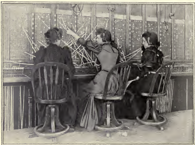
The Switchboard of a Telephone Exchange
